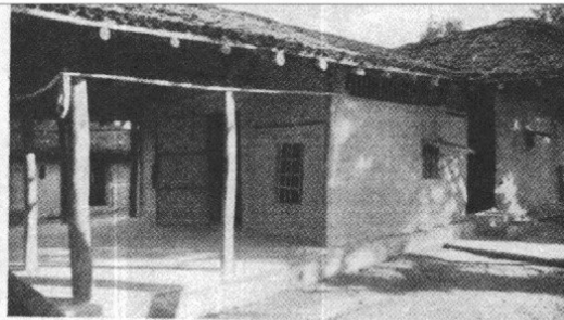
Figure 7. Close-up showing veranda, eaves ventilation and window screens Delia Tyrwhitt, London
